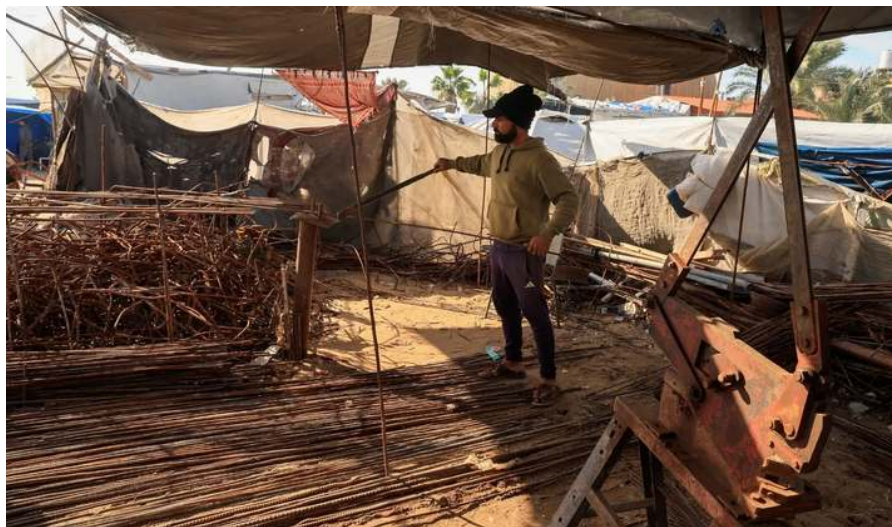
A Palestinian worker reshapes and straightens steel bars recovered from destroyed homes using basic tools inside a small workshop in Khan Younis, southern Gaza Strip, December 10, 2025. PHOTO CREDITS
