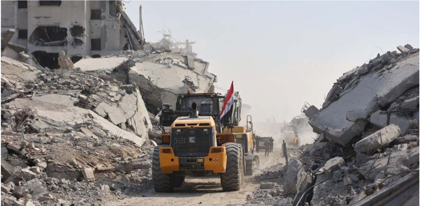
Construction equipment supplied by Egypt drives through Gaza City on November 2, 2025. PHOTO CREDITS
