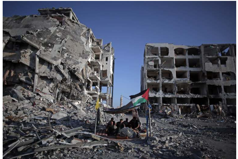
A group of Palestinians sit in a shelter made of a blanket stretched over four poles next to one of the destroyed Nada Towers in the Gaza Strip. PHOTO CREDITS
